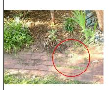
The front sidewalk has settled and is possibly causing a trip Hazard recommend repair
